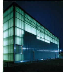
The translucent Rodeca cladding to the academy hall provides a skin that undercuts the mass of the hall, achieves internal daylight and at night produces what appears to be a shimmering, skeletal object.
