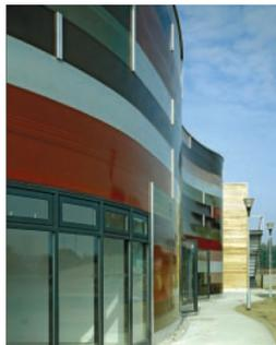
The use of horizontally paneled, multi-coloured polycarbonate cladding on the peanut responds to the desire to create a friendly, energetic and memorable building that lives up to its landmark status.
